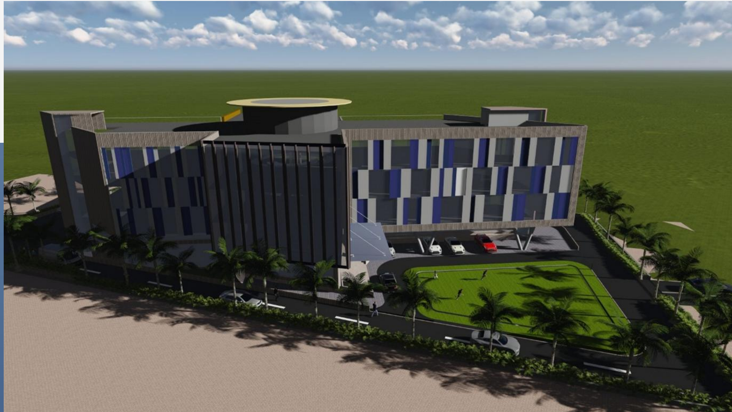
SCHOOL AT GURUGRAM Arch : Habitat Design Centre Area : 60,000 Sq.ft
